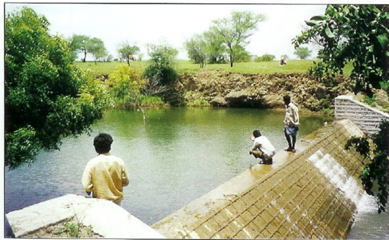
Figure 5. Community-based masonry check dam.
