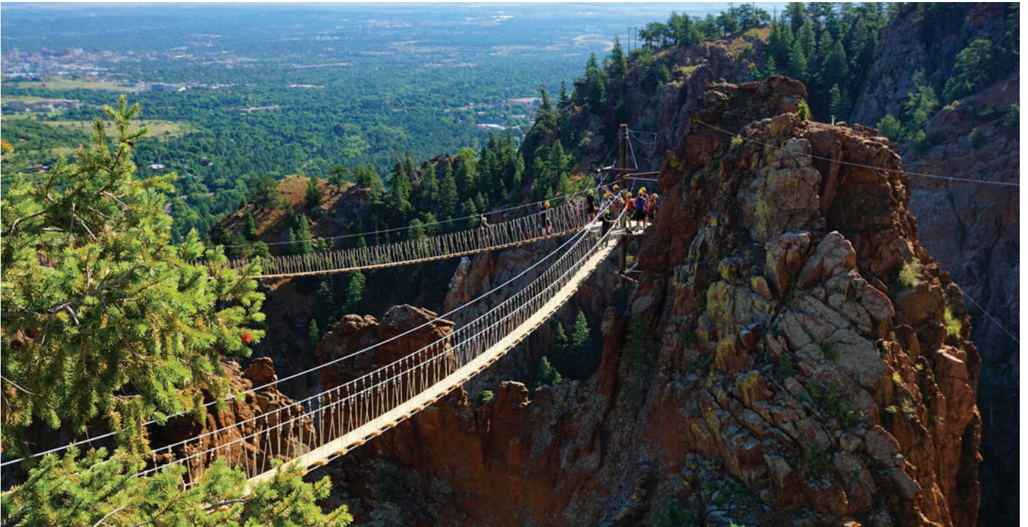
Terra-Flight Broadmoor Bridge Platform
