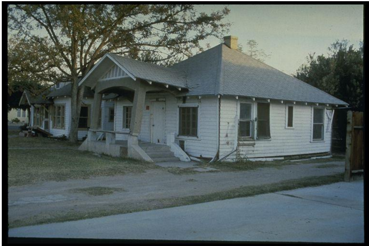
Figure 3–2. Image showing cripple wall collapse on a wood frame house in the 1979 Imperial Valley, California, earthquake.
