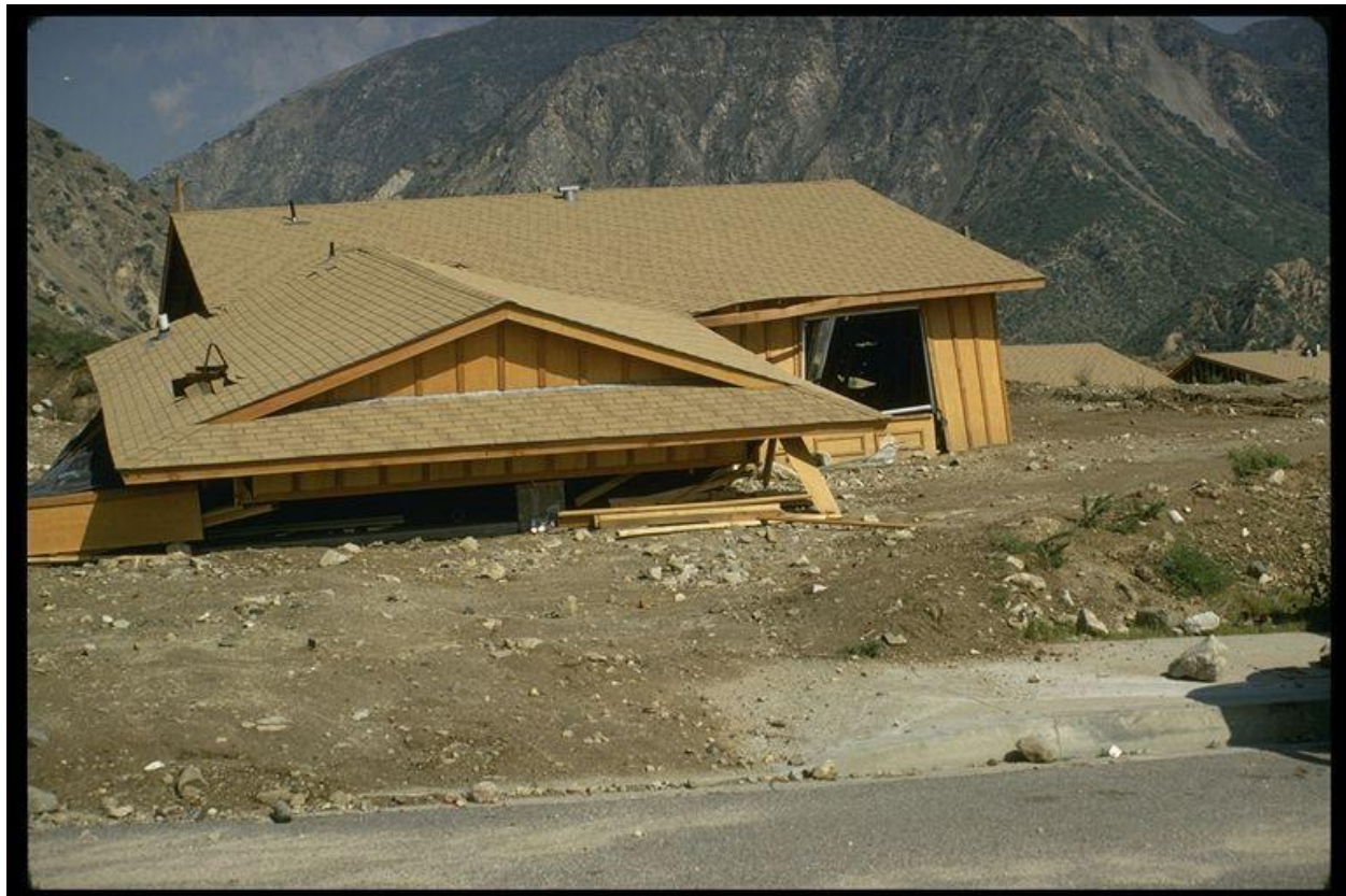
Figure 2-17. Image showing a collapsed wood frame house in the 1971 San Fernando, California, earthquake.
