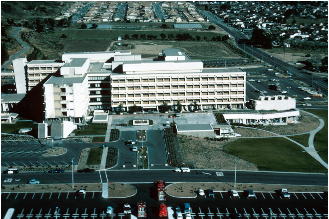
Figure 2–13. Image showing collapsed and leaning stair towers at Olive View Hospital, Sylmar, in the 1971 San Fernando, California, earthquake.
