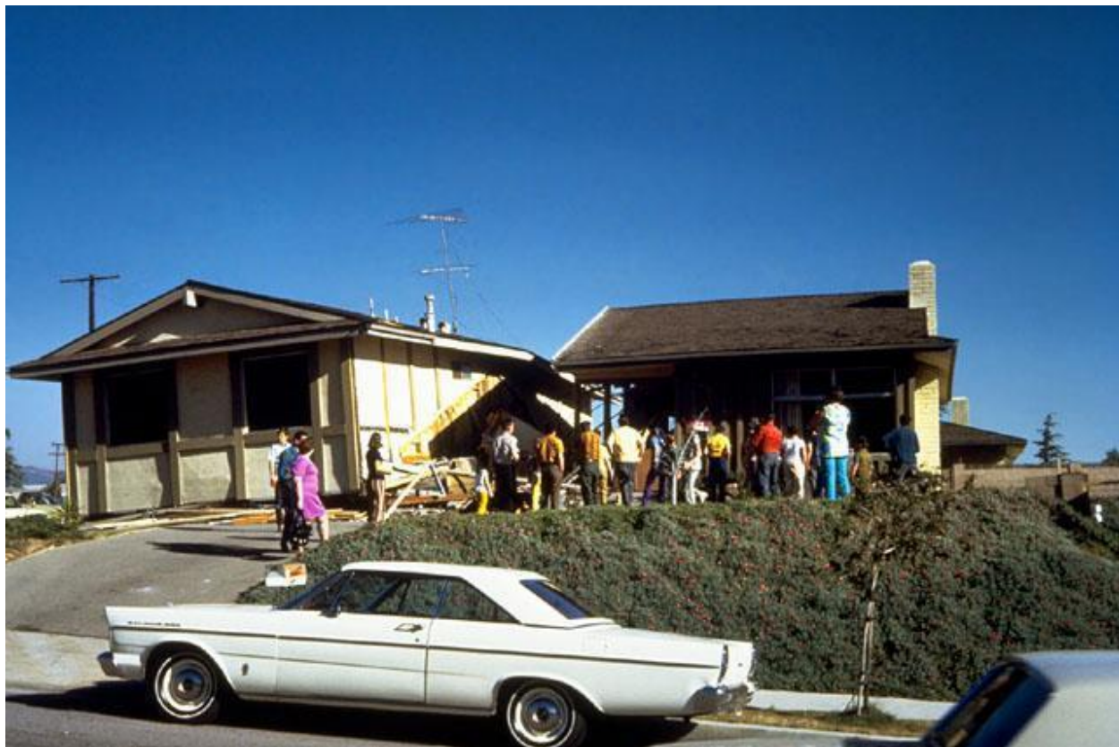
Figure 2–8. Image showing damage to a split-level house in the 1971 San Fernando, California, earthquake.
