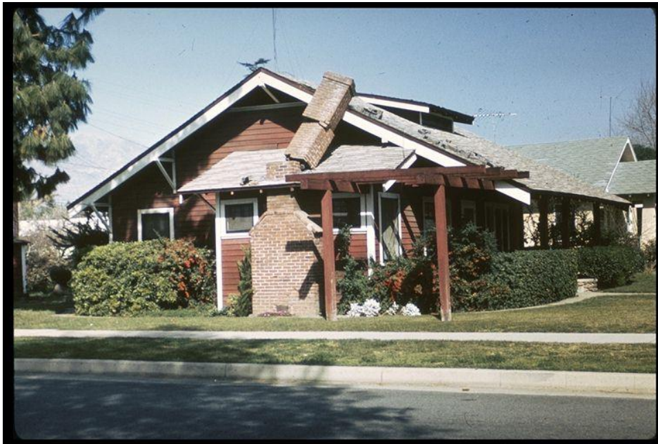
Figure 2-2. Image showing chimney damage in the 1971 San Fernando, California, earthquake.
