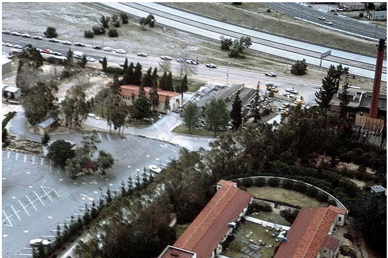
Figure 2–19. Image showing damage to the Veterans Administration Hospital, Sylmar, in the 1971 San Fernando, California, earthquake.
