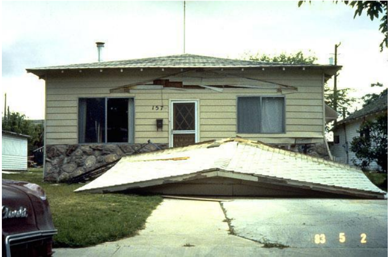
Figure 5-3. Image showing collapse of a wooden porch in the 1983 Coalinga, California, earthquake.
