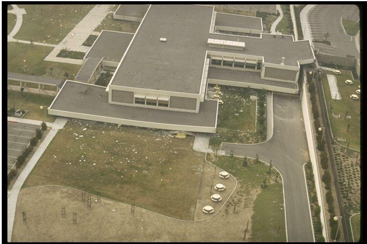
Figure 2–15. Image showing soft-story collapse of Psychiatric Building at Olive View Hospital, Sylmar, in the 1971 San Fernando, California, earthquake.
