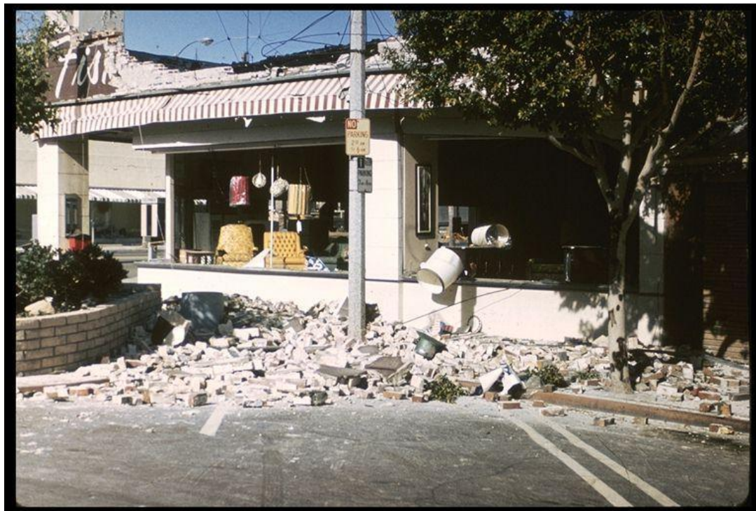
Figure 2-3. Image showing furniture store damage in the 1971 San Fernando, California, earthquake.
