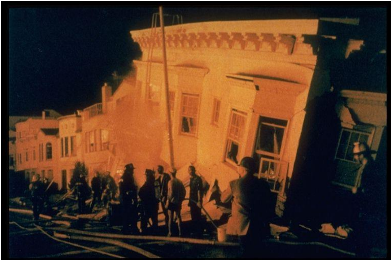
Figure 8–11. Image showing collapsed four-story building in the Marina District, San Francisco, in the 1989 Loma Prieta, California, earthquake. [Source: Scawthorn et al. 1992, p.204, fig. 11.]
