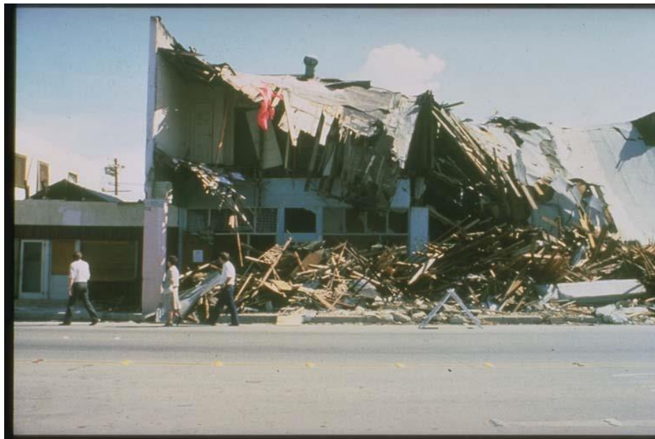
Figure 4-1. View of a two-story building on West Main St, Westmorland after the April 26, 1981 Westmorland earthquake
