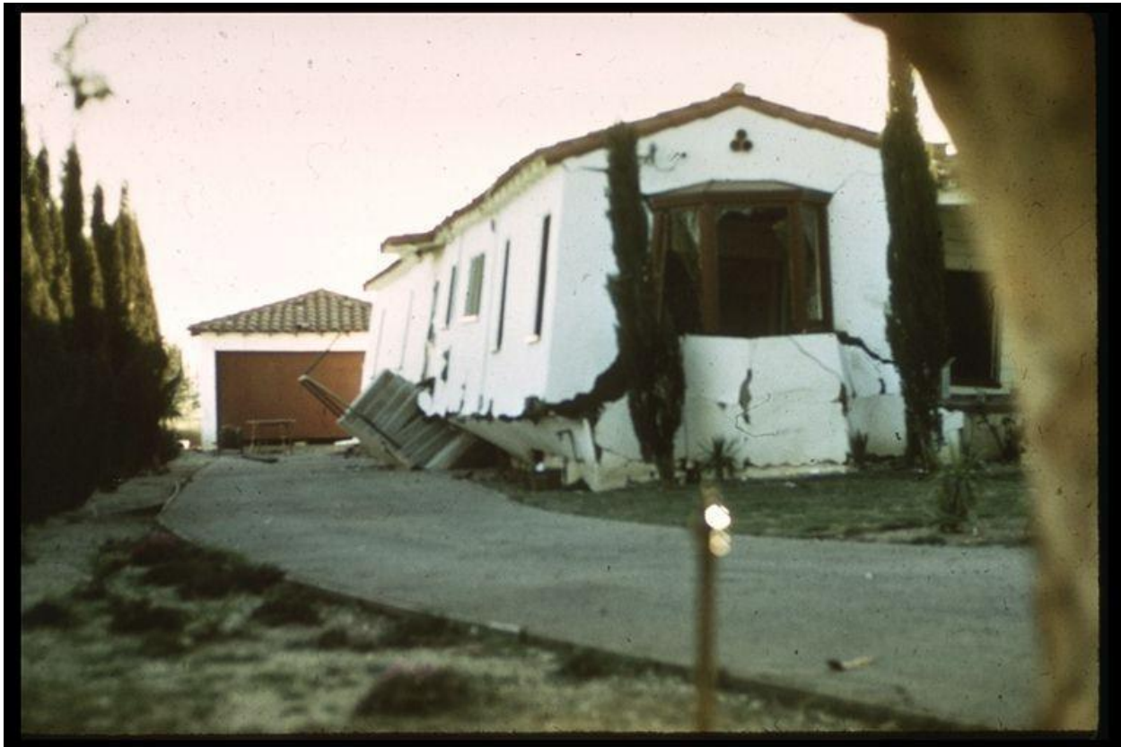
Figure 2–11. Image showing damage to older dwellings in the 1971 San Fernando, California, earthquake.
