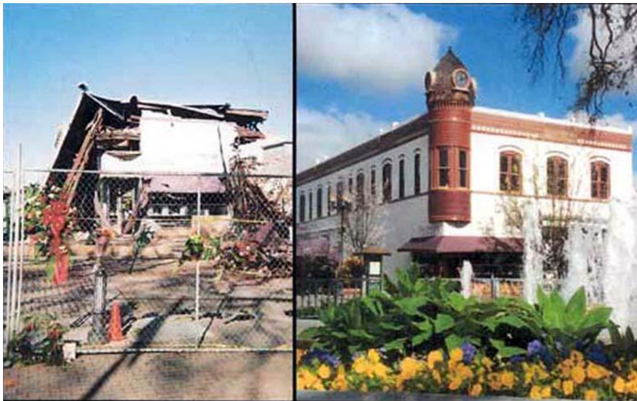
Figure 10–2. Before (right) and after (left) photographs of the Old Clock Tower, Paso Robles, in the 2003 San Simeon, California, earthquake. This unreinforced masonry building was built in 1892, and its clock tower had become a symbol of Paso Robles. The second story of the building collapsed directly westward onto Park Street.
