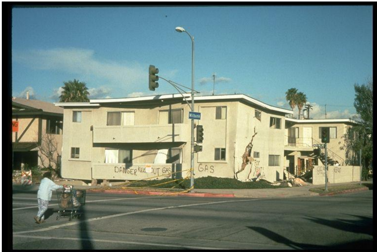
Figure 9–16. Image showing soft-story collapse of apartment building in Sherman Oaks in the 1994 Northridge, California, earthquake.
