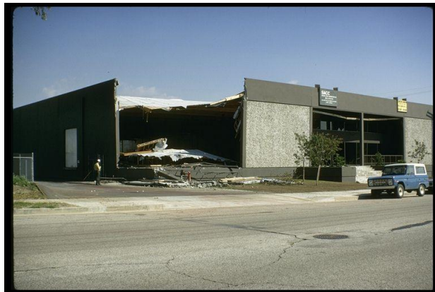
Figure 8. Example of both modal and median collapse of tilt-up. Photo credit: V. Bertero, courtesy of the National Information Service for Earthquake Engineering, PEER-NISEE, University of California, Berkeley.
