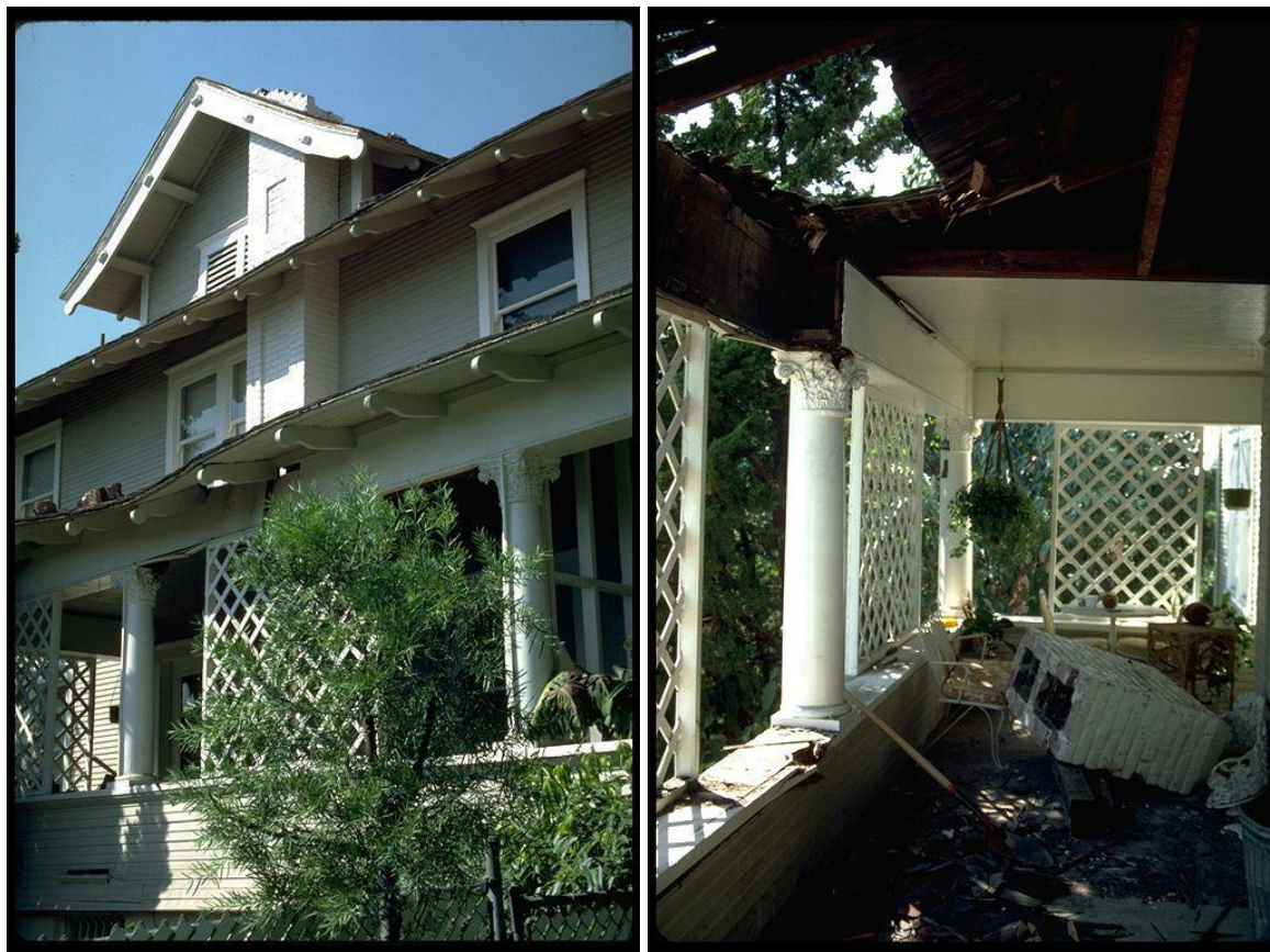
Figure 7-3. Image showing collapsed chimney in the 1987 Whittier Narrows, California, earthquake.
