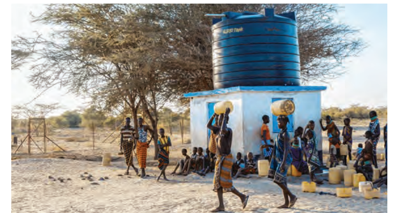
A groundwater pump station in Turkana, Kenya.
