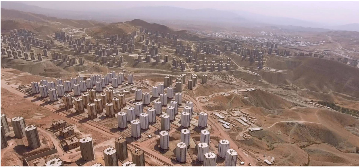
A modern housing development outside of Tehran, Iran. Kuzu Grup.
