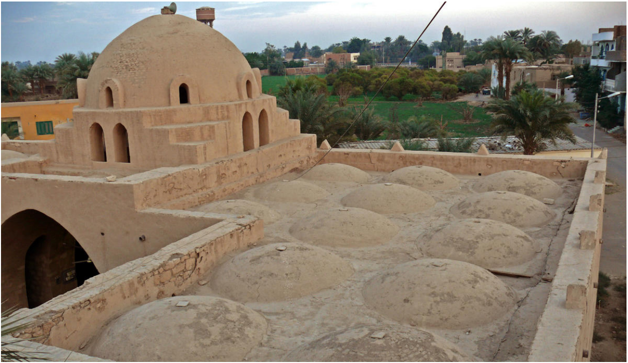
The roof of New Gourna's mosque. WMF.
