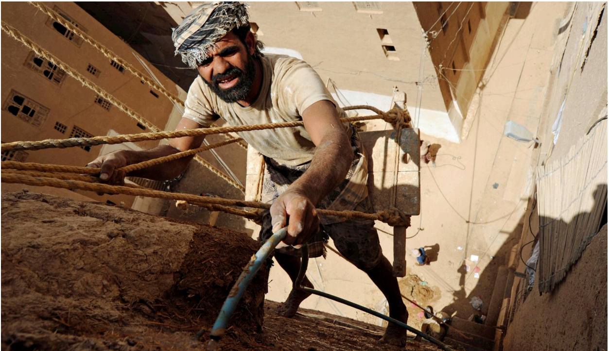
A man repairs a wall in Shibam. Ullstein Bild.
