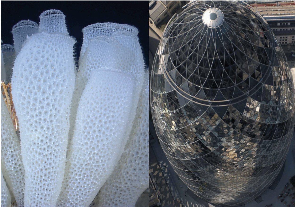
Figure 6: Venus' flower basket ( Euplectella aspergillum ) influenced the design of 30 St. Mary London, United Kingdom. Venus' flower basket ( Euplectella aspergillum ) [left] and 30 St. Mary [right]. (Sources: https://asknature.org/strategy/silica-skeleton-is-tough-and-stable/ & http://www.harvarddesignmagazine.org/issues/35/30-st-mary-axe )
