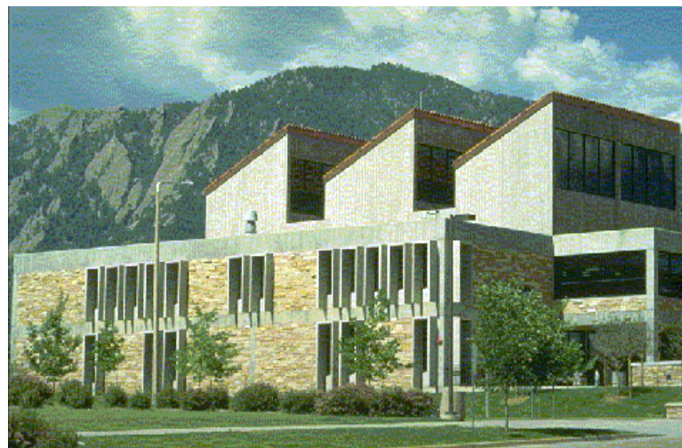
Figure 8.32. The Integrated Teaching and Learning Laboratory (1997) connects with the Engineering Center to the west. It was named the Grand Prize Winner for buildings built in Colorado by the Construction Management Report in 1997.
