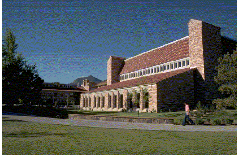
Figure 8.27. This addition to Norlin Library was built in 1977.
