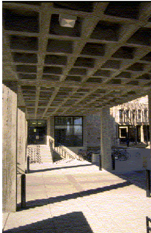
Figure 8.38. The square “waffle” pattern under the bridge saves weight.
