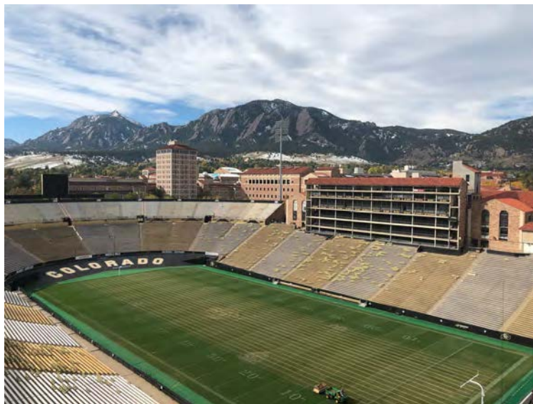
View from the Folsom Field Rooftop Terrace
