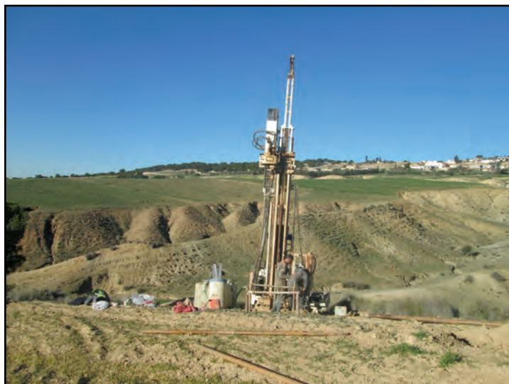
Drilling in El Kef, Tunisia (credit: H. Negra)
