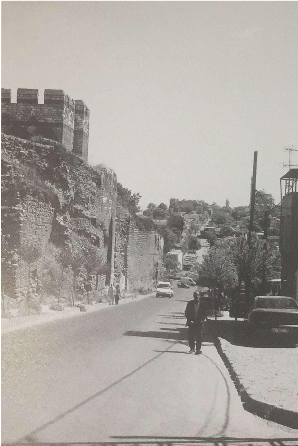
Figure 10 Elevation drop at the 5th Military Gate/ Gate of Saint Romanus (Philippedes and Hanak, Plate 66).
