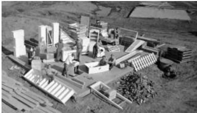
Figure 4. Workmen and the materials to construct a house gathered in a lot before construction, June, 1948. Photograph taken by Tony Linck for *Life*. Image from Hales, "Building Levittown."
