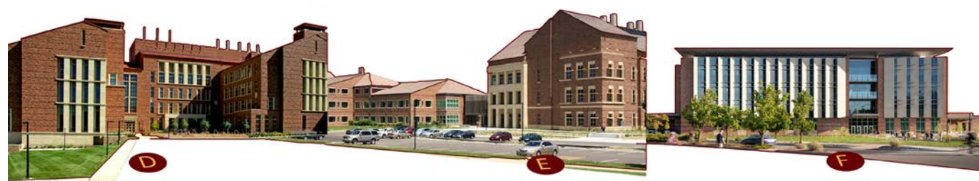
District character of East Campus
