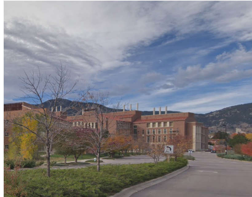
Existing View Along Discovery Drive
