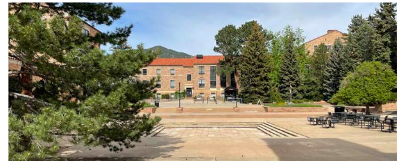
Existing Conditions at Trumbo Fountain
