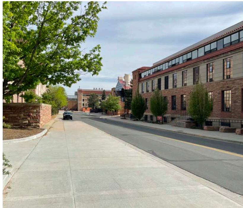
Existing Conditions looking North along 18th street
