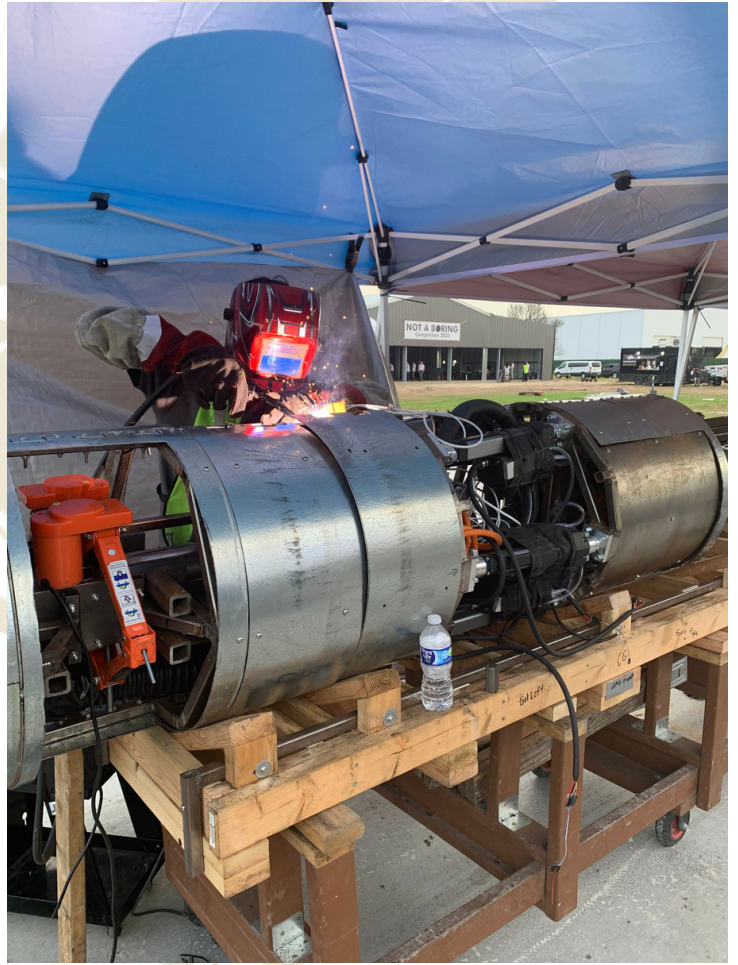
Arjun welding some modified gripper structures to the machine on-site
